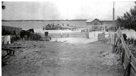
View from Gidneys house to jetty.
