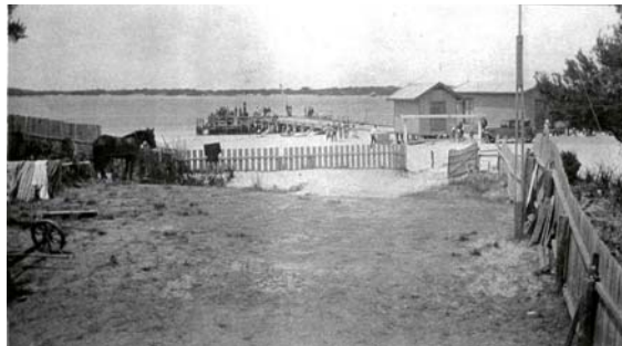
View from Gidneys house to jetty.
